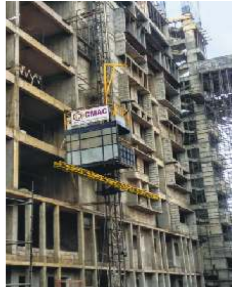
PM Hoist with 12mts Horizontal rebar carrier
