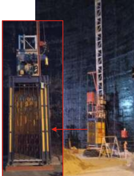
Chimney Hoist Yadadri Power Project, TS.
