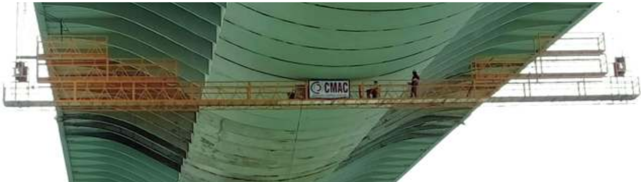
Bridge Special SRP at Durgam Cheruvu, Cable Stayed Bridge, Hyd.
