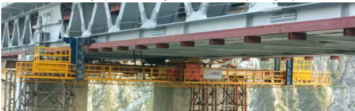
ANJI KHAD CABLE STAYED BRIDGE PROJECT, Dist.: Reasi, Jammu
